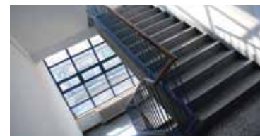
Internal works on housing property
